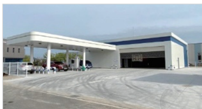
▲ Hydrogen Charging Station
