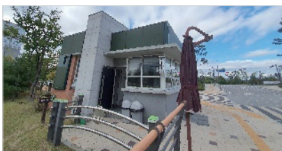
▲ Building Integrated Photovoltaic System (BIPV)
